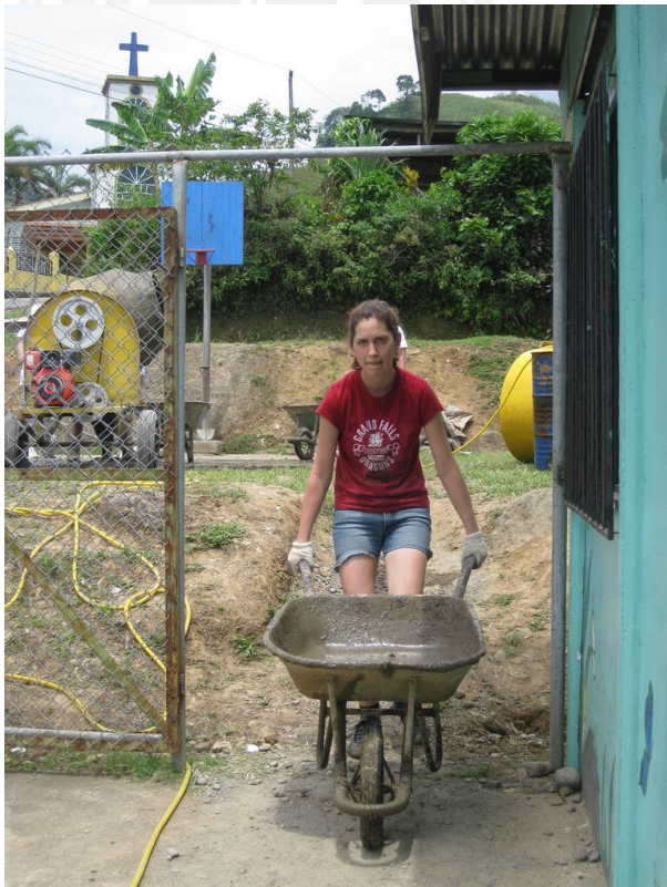
Moving cement for the library foundation.
