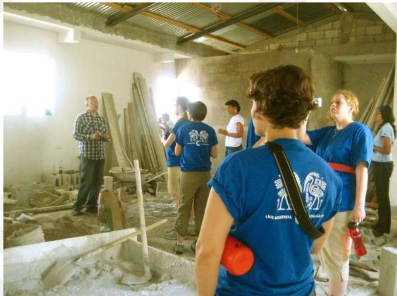
Getting a tour of the new library under construction.
