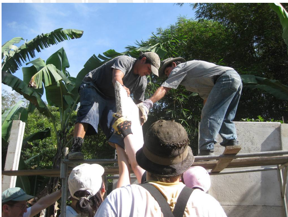
Raising the walls of the new library.
